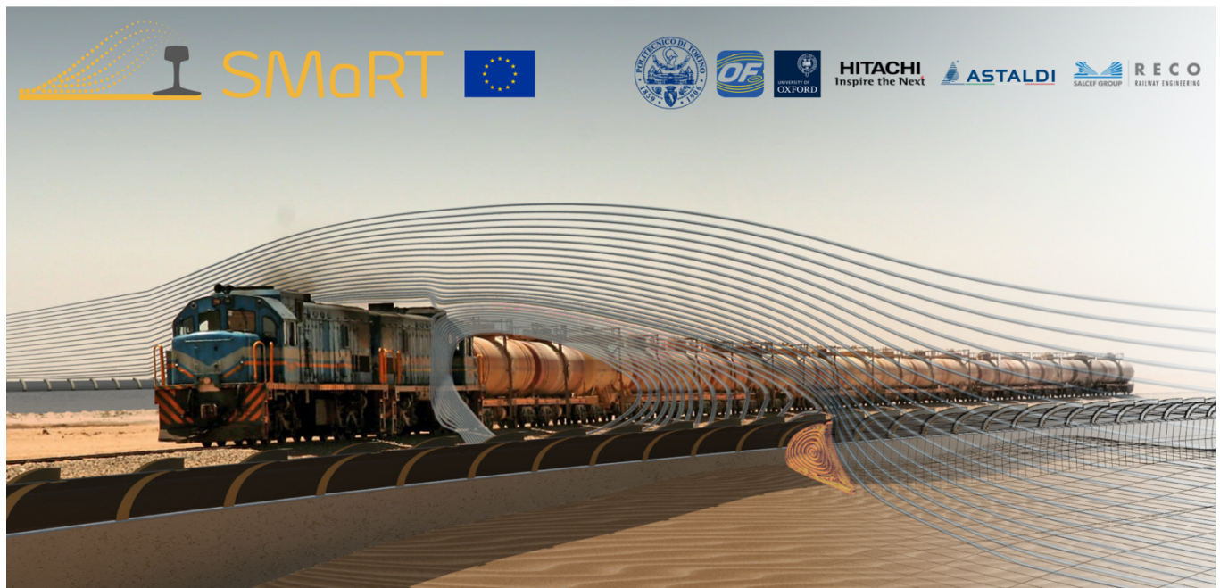
Example of a Sand Mitigation Measure and its aerodynamic working principle
