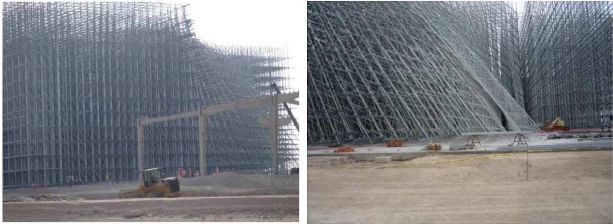
Figure 1. Partial collapse of an ARSW during construction phase.
