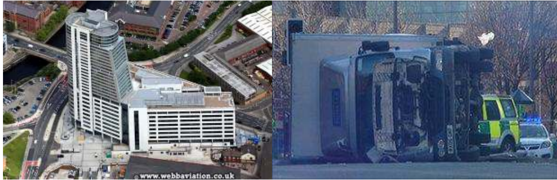
Figure 1. Bridgewater Place in Leeds UK and the accident of March 2011
