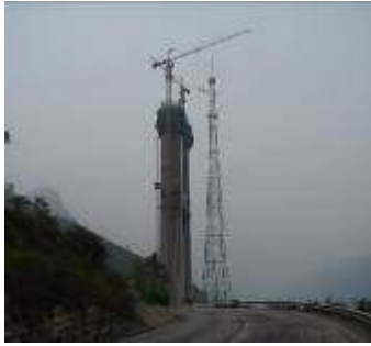
Figure 3 Observation Tower at the Bridge Site
