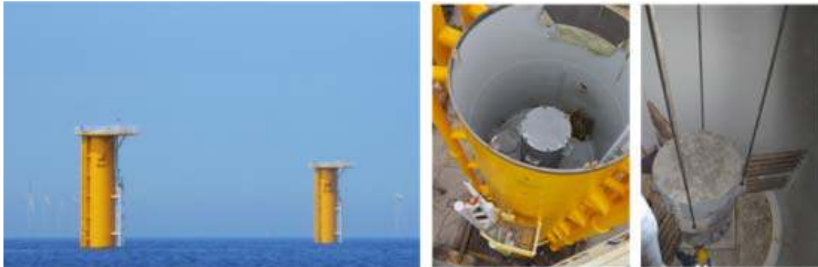
Figure 10. Passive Tuned Mass Damper applied at a transition piece to reduce wave induced vibrations
