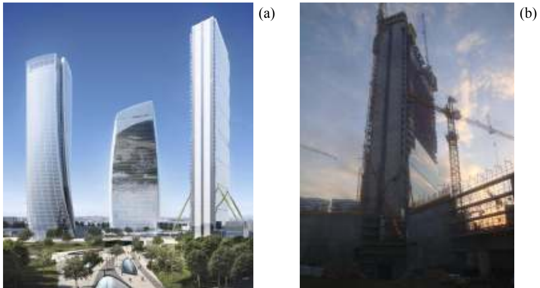
Figure 1. Perspective view of the masterplan of the new business and shopping district of CityLife in Milan, Italy with Isozaki tower on the right (a); the Isozaki tower under construction (b).
