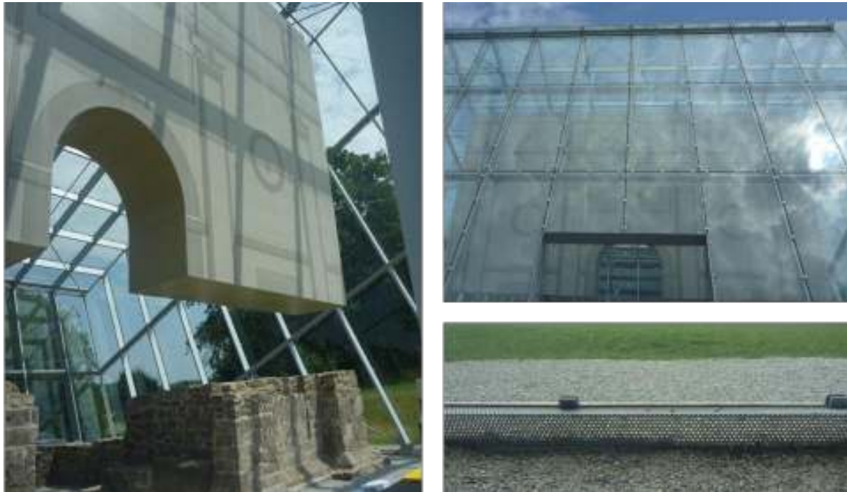
Figure 2. Internal views: the plastic replica of the ancient Roman gate (a). Openings at the top of the southern façade (b) and at the bottom of the entire perimeter (c).
