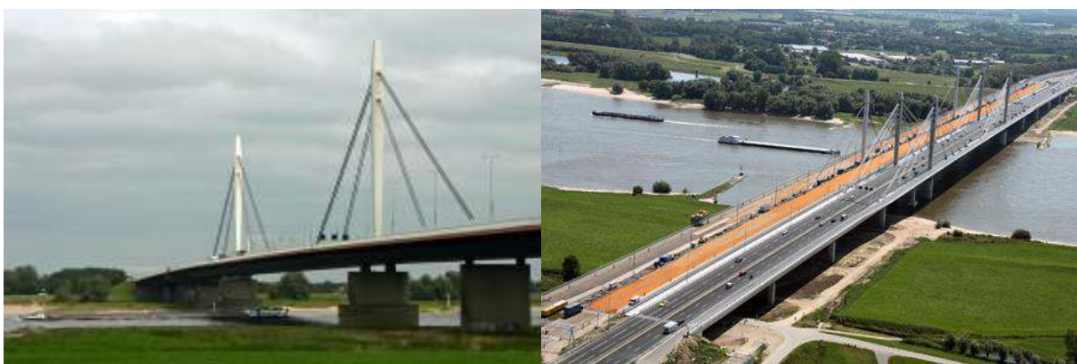
Figure 1. The Ewijk Bridge. On the left: original stand-alone configuration. On the right: the new configuration with the existing deck (in refurbishment) and the new deck.
