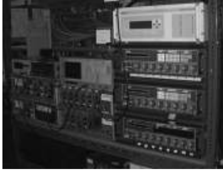
Figure 4.18 External amplifiers for pressure sensors type 1
