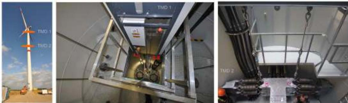
Figure 11. Tuned Mass Damper for Mode1 and Mode 2 of a wind turbine tower
